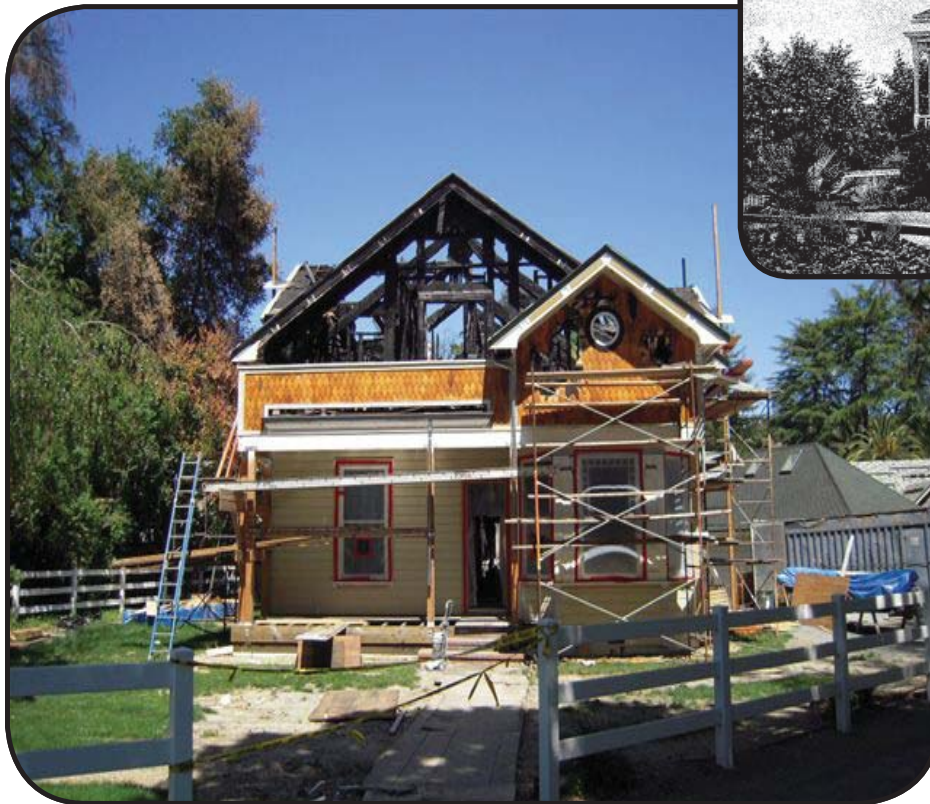
Historical home under renovation.
